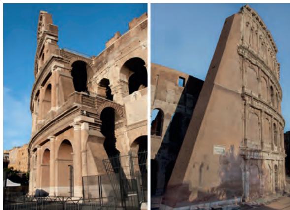
Fig. 5 Rome, Parco archeologico del Colosseo. Colosseum. Counterforts by Stern and Valadier in detail.
