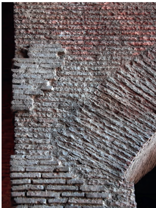
Fig. 8 Rome, Parco archeologico del Colosseo. Forum Romanum, Santa Maria Antiqua. Detail of the pounded brickwork compared to the original masonry.
